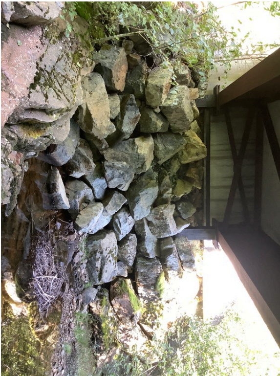
Left Bank Abutment when facing downstream
